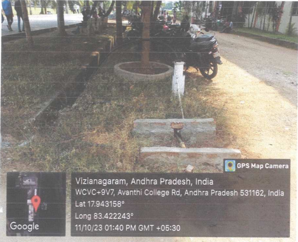
Bore well in front of AIPS campus
