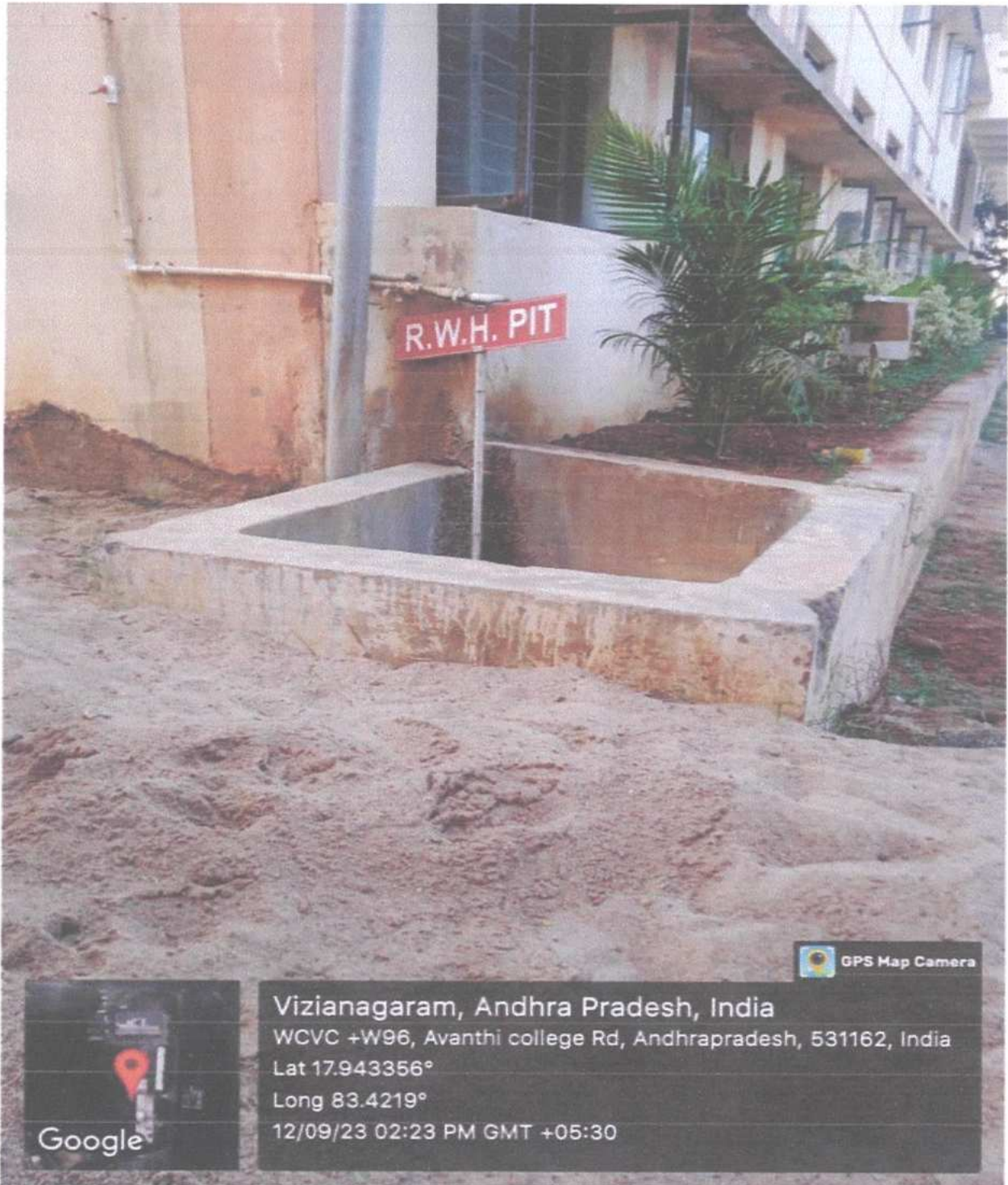
Rain water harvesting pit at AIPS campus for water conservation
