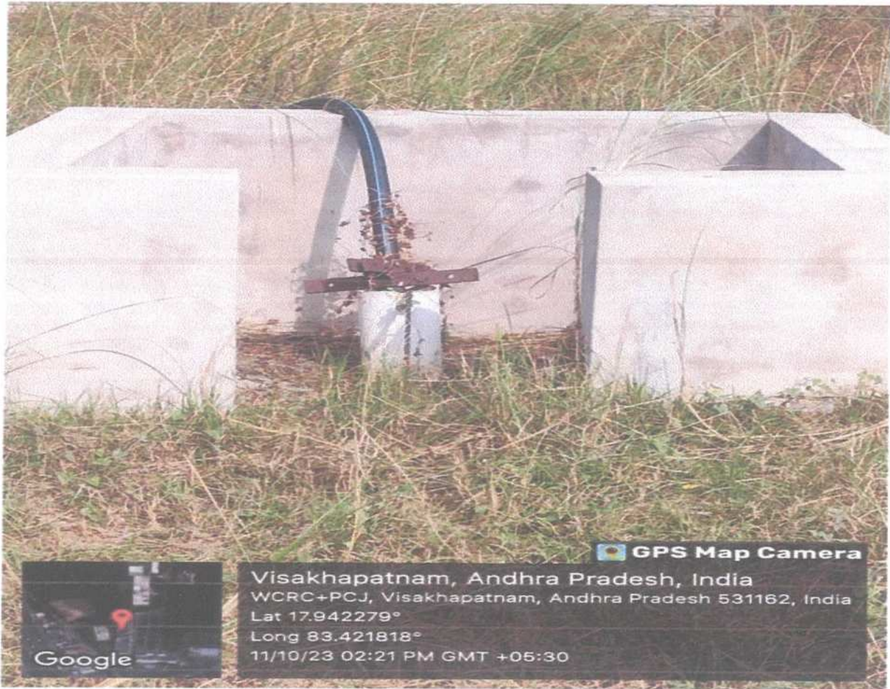
Bore well installed in the rear area of the pharmacy block
